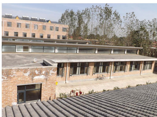
Renovation project of Liming Youth Rehabilitation Centre, Tongqiu town, Hebei province
